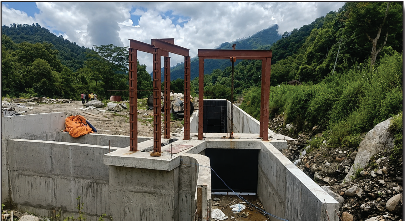
Cascade Headpond and Diversion Structure
